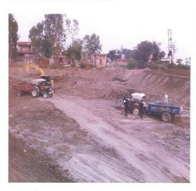
First the existing pond was drained out in near by vacant land, and then the emptied pond was de-silted. It was then divided into four compartments through earthen embankments. The village drain is led into the first compartment. The overflow goes in to second compartment and then to the third and the fourth tank.
