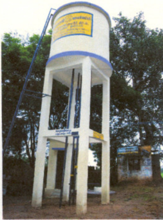
COMPLETION STAGE - 10,000 LITRES CAPACITY OHT
