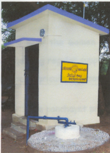
COMPLETION STAGE - SOURCE AND PUMP ROOM
