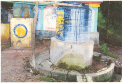
EXISTING WATER SUPPLY SYSTEM - MINI POWER PUMP
