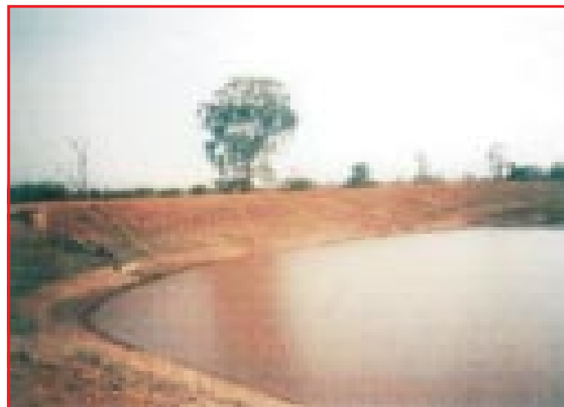
Restoration of Bhandar Tank Head Works in Kabirdham district of Chhattisgarh
