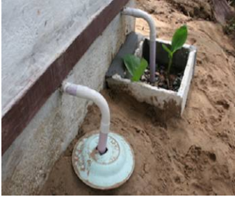
Arrangements for collection of urine and wash water
