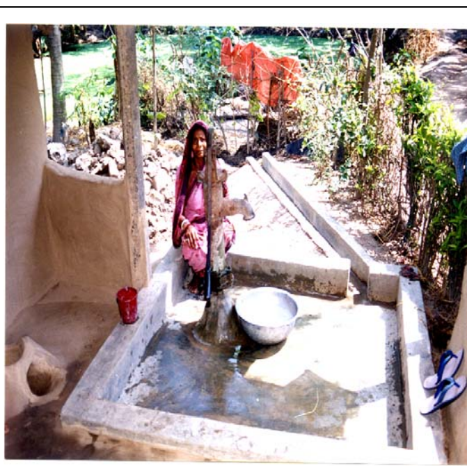
Hand Pump with Platform and Darin
