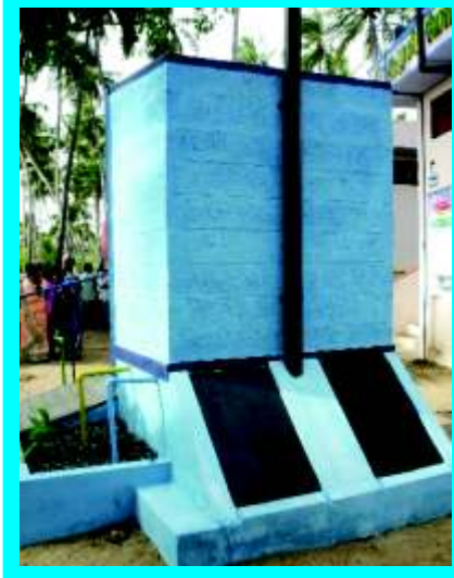
Ecosan Toilet Using Solar Energy
