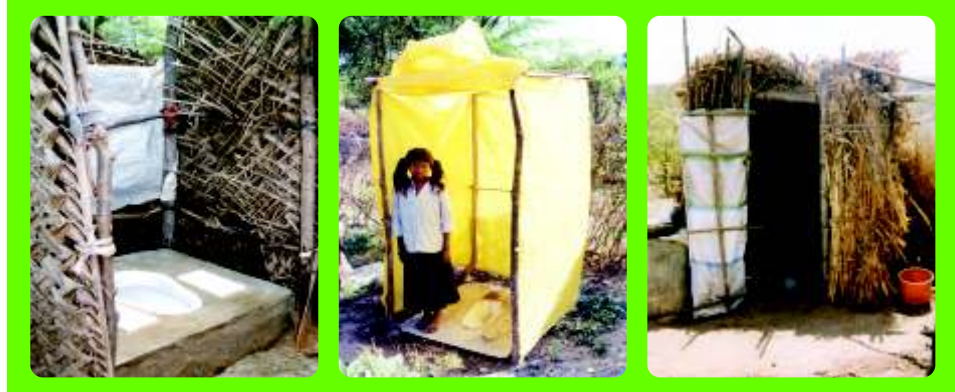
Leach pit latrines with steep pan with seal of only 10-20 mm
