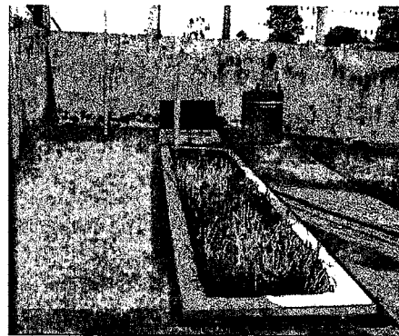
Fig: BioTank cum Reed Bed system: in this fig., biotank is horizontally separated by an incomplete partition wall. The water from the biotank, (after travelling the long path) is released into reed bed. The water from the reed bed may be stored to a tank for further use or may be released directly to the agro fields for irrigation.
