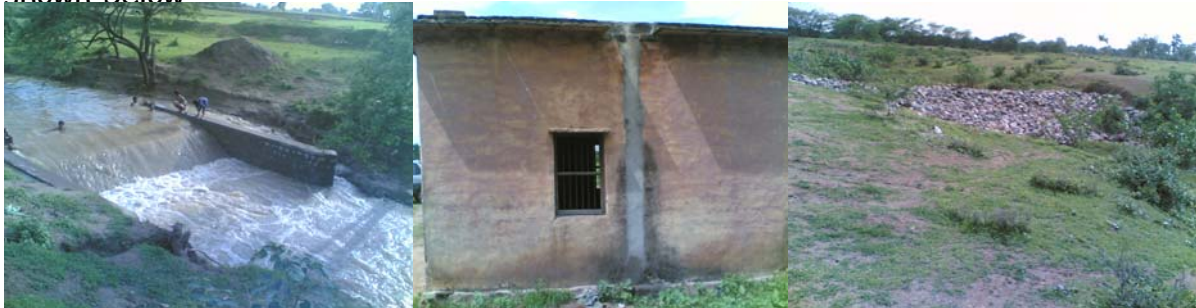
Check-dam constructed by PHED
