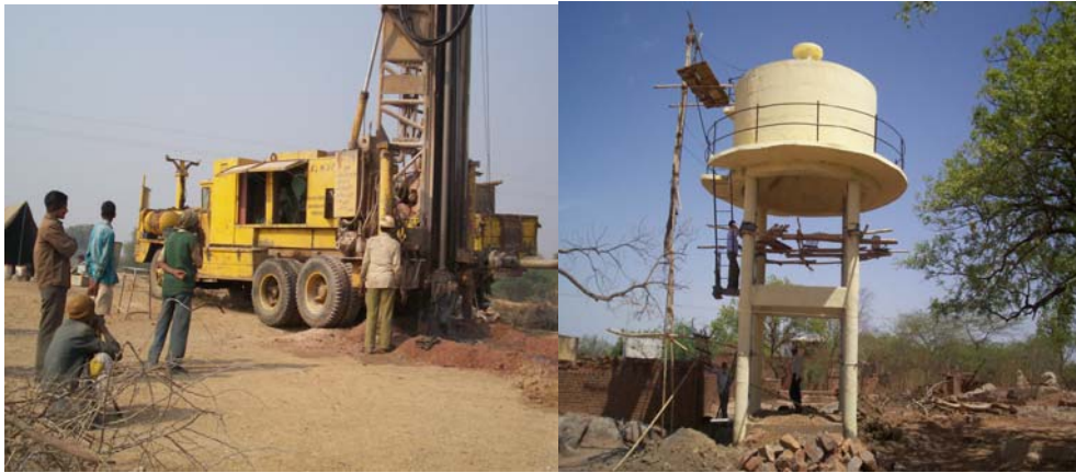
VWSC initiated construction of a new Mini Water Supply Scheme
