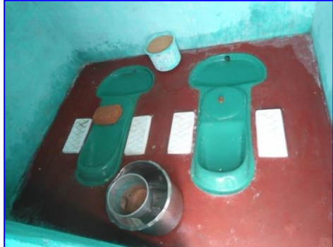
Inner View of ECOSAN UDDT
