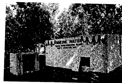
Terafil water purification plant (30,000 Lit/day capacity)
