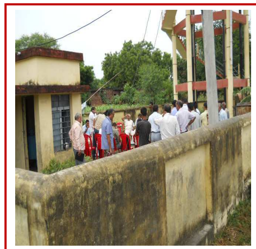
Deep Tube-well based Piped water supply
