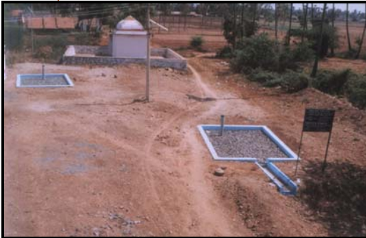
The shaft is provided with a reverse drainage that facilitate intake of stored water from the pond through a narrow raised channel with a metal filter to filter coarse materials.
