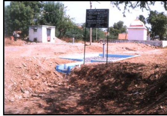
Pump room with functioning borewell, newly provided recharge shaft, storage pond and the display board scheme details.
