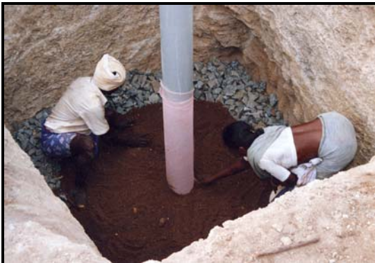
1*1*1.5 The telescopic trench and the newly inserted perforated PVC casing pipe.
