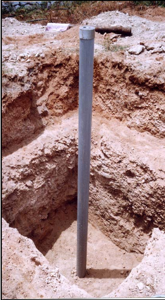
1*1*1.5 The telescopic trench and the newly inserted perforated PVC casing pipe.
