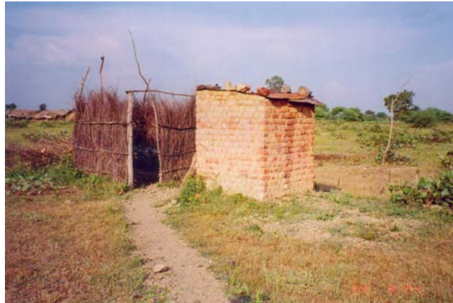
Photo: 22 A well maintained household toilet with brick super structure of a BPL beneficiary. Village Khokhri, Problem of Water logging is faced during rainy season. (Sehore)
