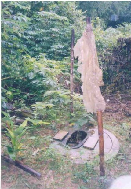
Photo: 25 Under utilized Toilet at Borda Village (Medinipur West)
