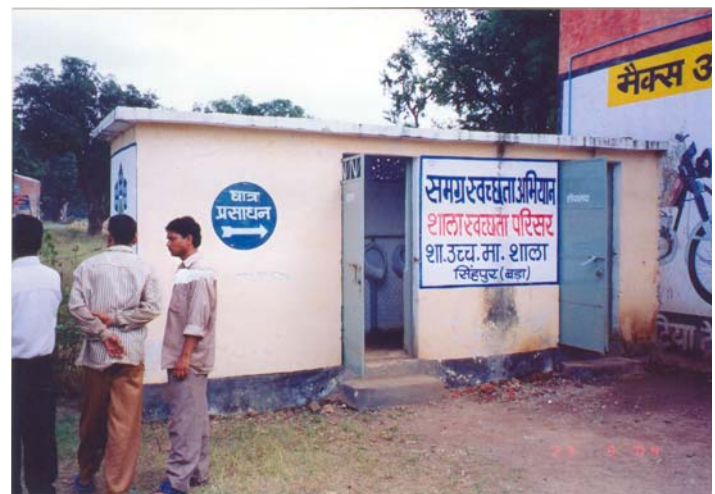
Photo: 29 Well maintained School toilet at Government Senior Secondary School, Village Singhpur. (Narsinghpur)
