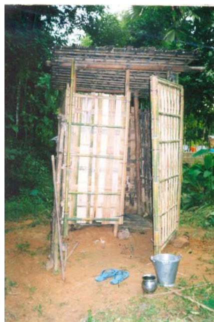
Photo: 20 Individual Household Latrine with super structure made of locally available material at South Maharani Village (Medinipur West)
